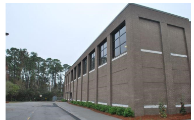
Coastal Middle Gym Addition
